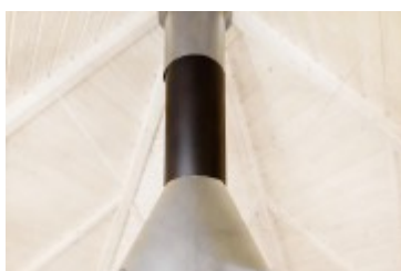
Grill Chimney Extension
